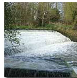
Sutton Hall Weir
