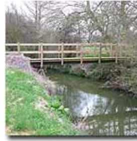
Footbridge over the River Uck at Little Horsted
