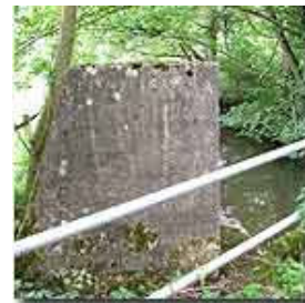
WW2 tank trap beside the River Ouse nr Slaugham Common
